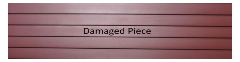
• Using a hand saw equipped with a continuous rim diamond tile blade, cut the entire length of the damaged piece of siding as close to the top as possible.
