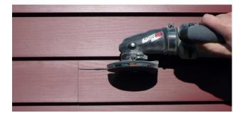
• Once the piece is cut, remove the bottom of the damaged part.
